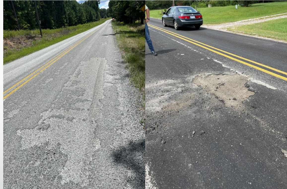
Poor Chip Seal
